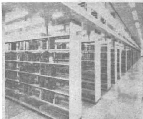
Multi-tier bookshelves and mezzanine cellular decking installed in September, 1964 at University of Victoria, B.C. Mr. Dean W. Halliwell, Chief Librarian, R. W. Siddall Associates, Victoria, B.C., Architect
