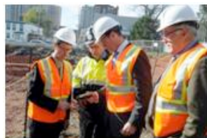
Minister MacKay, Minister MacDonell, Mayor Kelly and Terry Gallagher, manager of Infrastructure & Facility Development for HRM prepare to take a tour of the site
