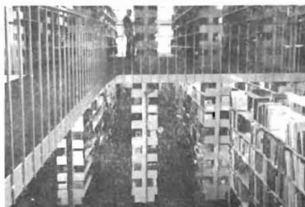
Library, Pavillon Lalemant, Collège Jean de Brébeuf, Montreal. This photograph shows how a Montel Mezzanine doubles useful shelving space in a high ceiling library — approx. 14 ft.
