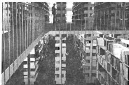
Library, Pavillon Lalemant, College Jean de Brébeuf, Montreal. This photograph shows how a Montel Mezzanine doubles useful shelving space in a high ceiling library — approx. 14 ft.
