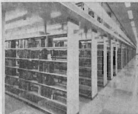
Multi-tier bookshelves and mezzanine cellular decking installed in September, 1964 at University of Victoria, B.C. Mr. Dean W. Halliwell, Chief Librarian. R. W. Siddall Associates, Victoria, B.C., Architect
